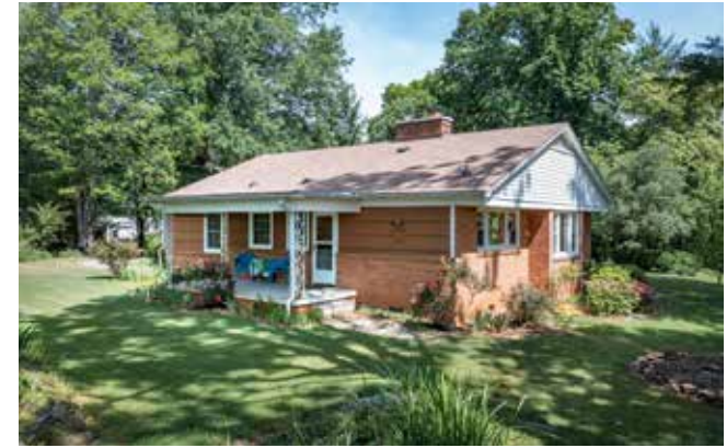
Side Porch with Mountain Views
