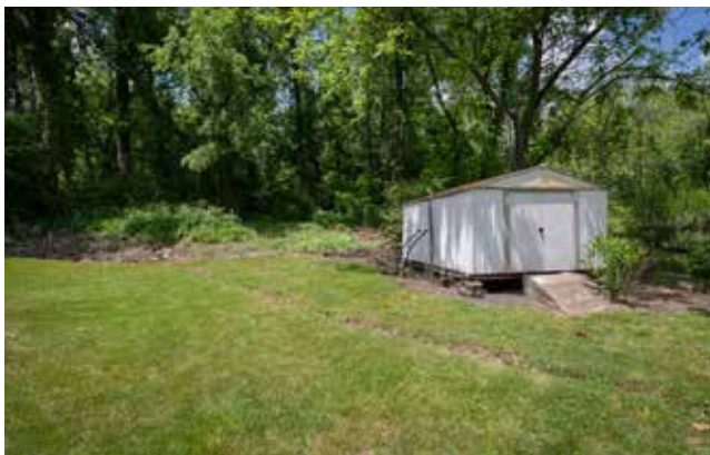
Shed for Additional Storage
