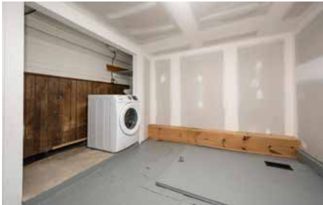
Laundry Room and Entrance to Crawl Space
