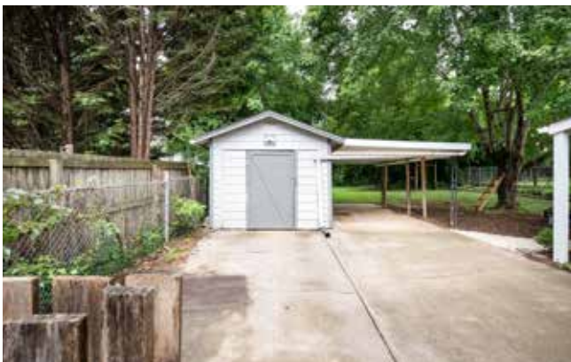
Workshop/Shed with Electricity and ...
