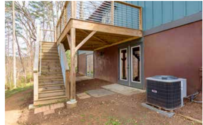
Newer Deck and Covered Back Patio
