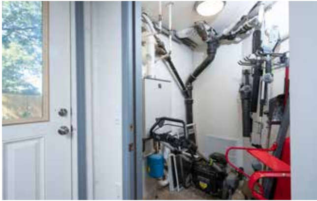
Even More Space for Storage Near the Back Door
