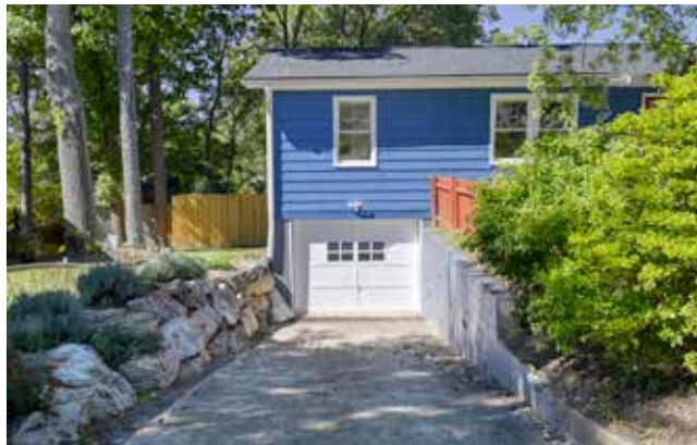
One-Car Garage for Parking, Workshop, and Storage
