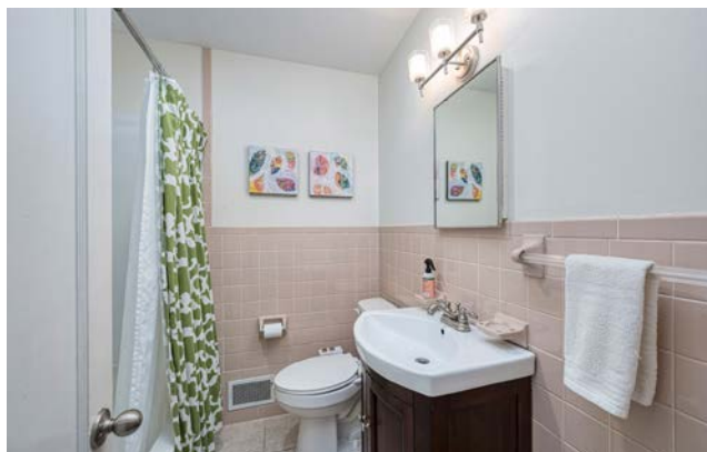
Original Tile with Updated Tub Surround and Fixtures
