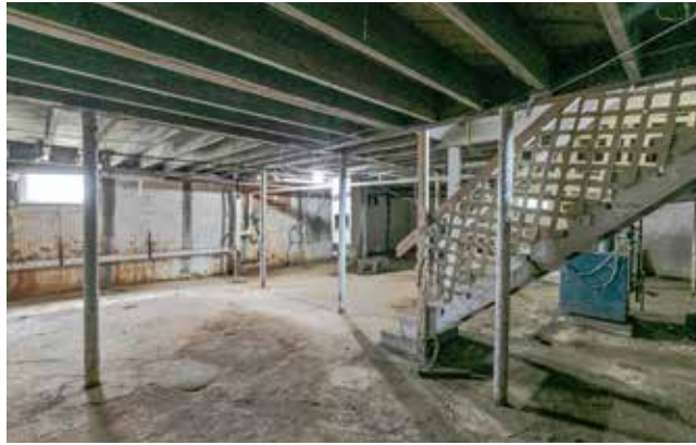
Expansive Unfinished Basement
