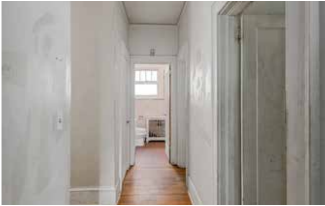
Hallway Connects Three Bedrooms on Main Level
