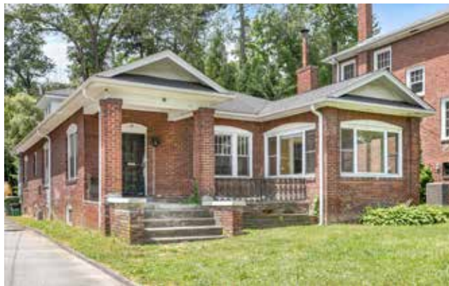
Full-Brick Exterior and Arched Lintels
