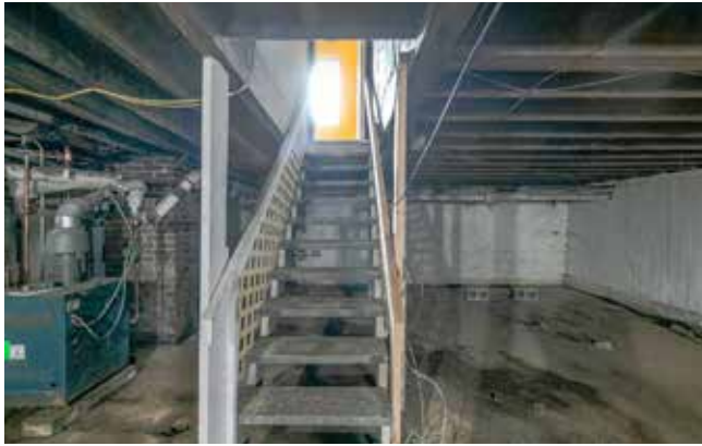
Interior Basement Access
