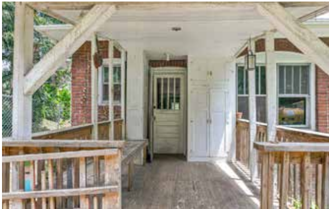
Covered Back Deck with Built-in Storage
