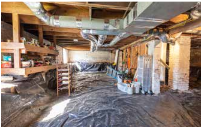
Stand-Up Crawl Space with Storage
