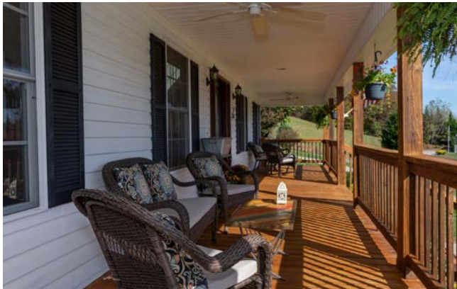
Recently Stained Porches
