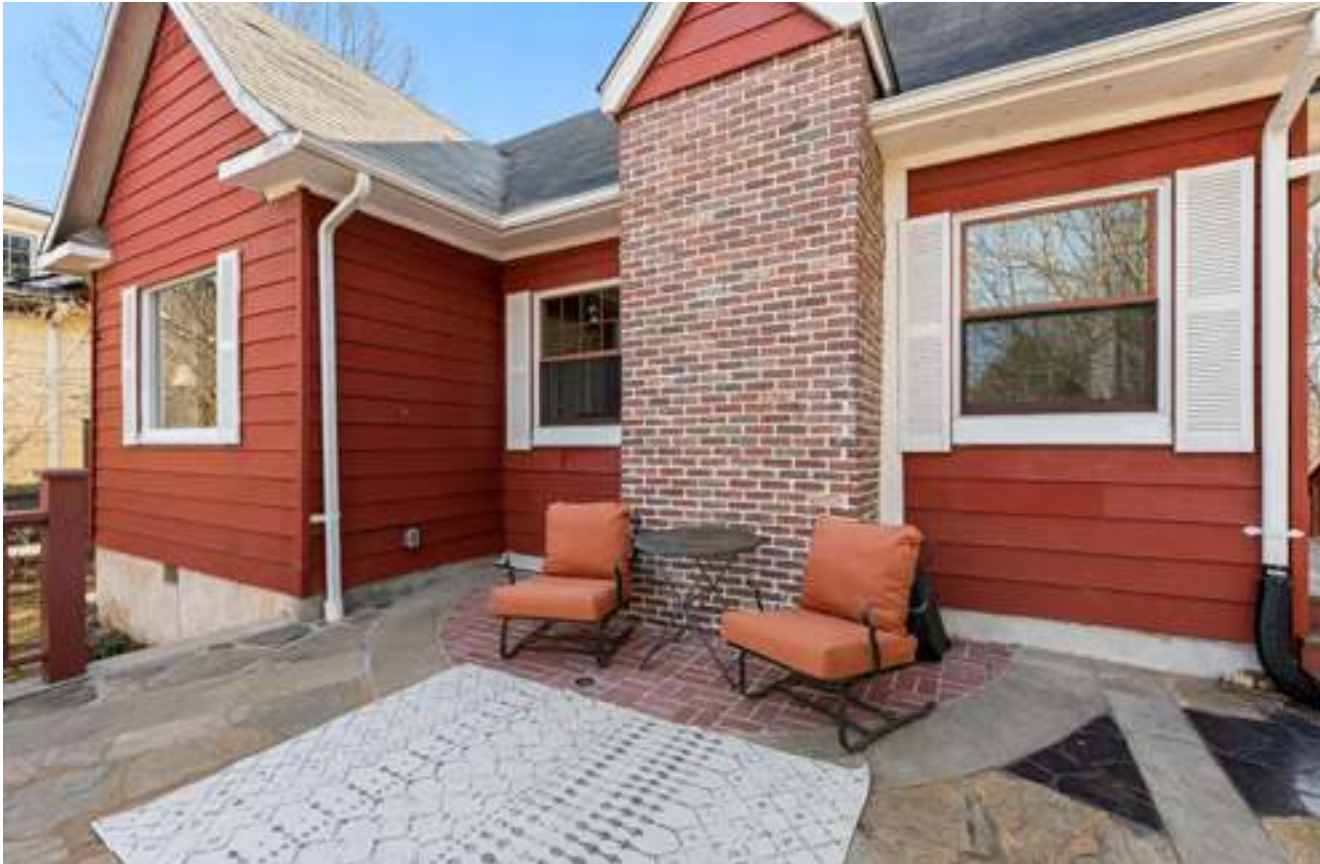
Reconstructed Chimney and Front Patio
