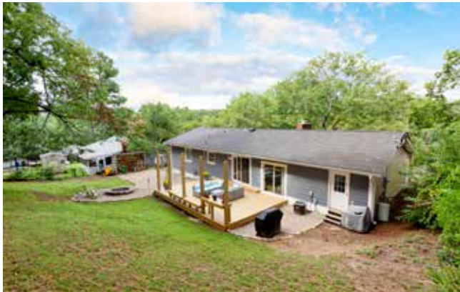
Access Deck/Back Yard from Dining Area and Primary Suite
