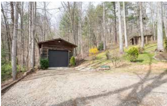
Detached One-Car Garage (Electrical Installed)
