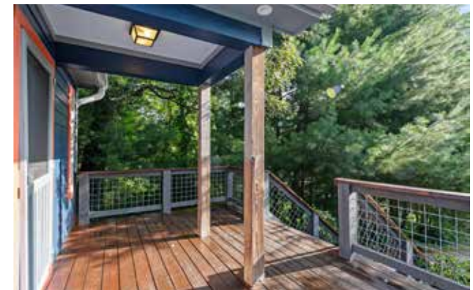
Covered Entryway on Large Front Porch
