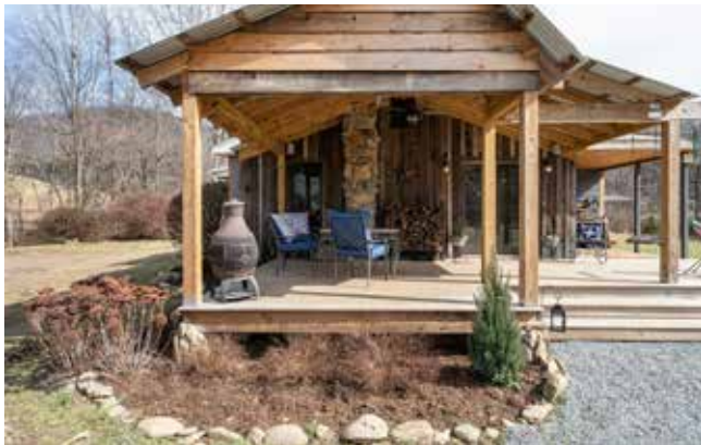
Covered Side Porch Leads to Indoor Dining Area
