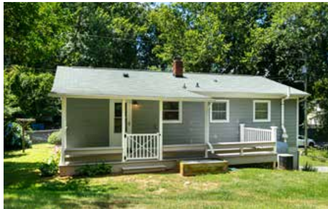
Radon System Installed, Note the Vent to the Right
