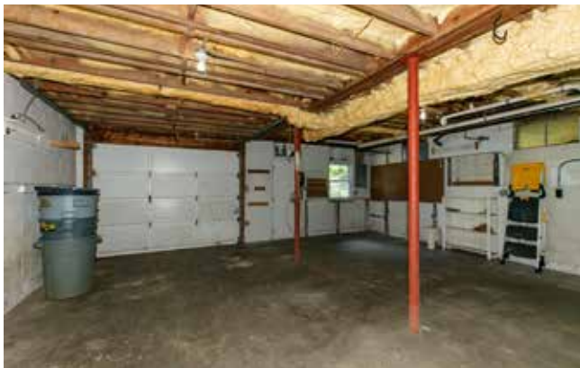
Single Garage/Basement Flex Space with Foam Insulation
