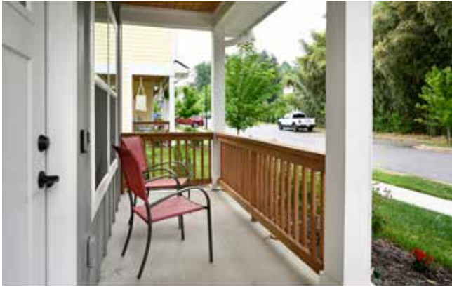
Covered Front Porch
