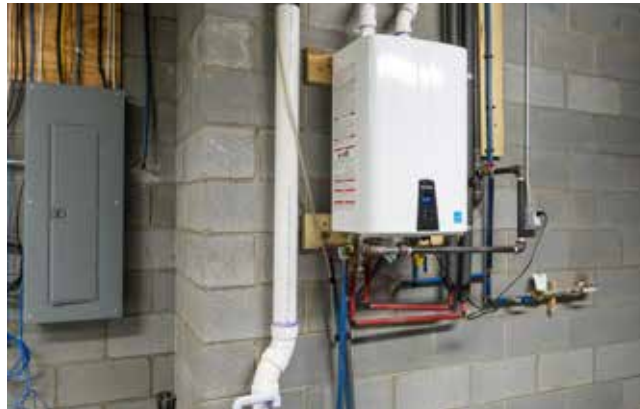
Tankless Natural Gas Water Heater
