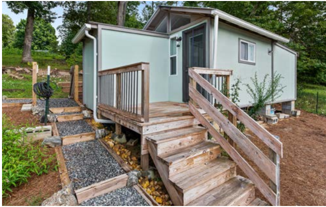
Side Entrance of Finished Shed
