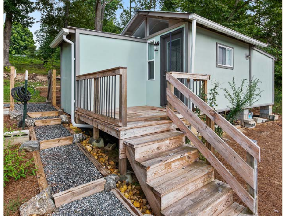
Hey, Cutie! Side Porch of Finished Shed
