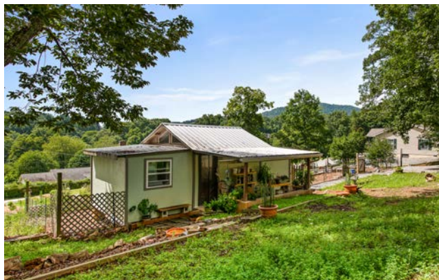
View of the Front of the Finished Shed
