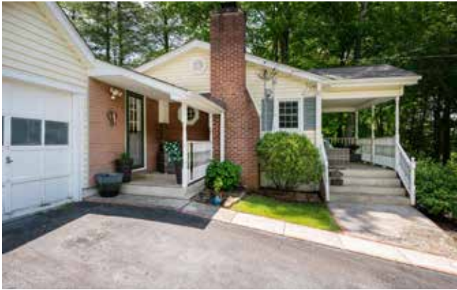
Two Front Accesses from the Covered Porches
