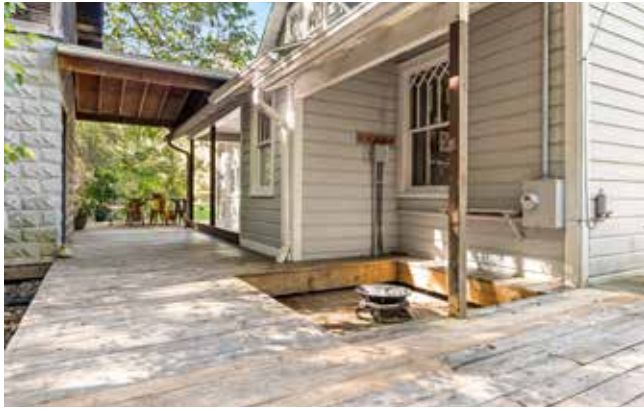
Large Back Patio and Deck
