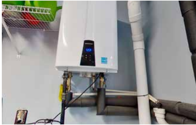
Natural Gas Tankless Water Heater
