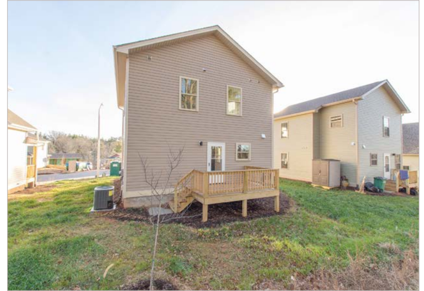
Back Deck Overlooks Green Space
