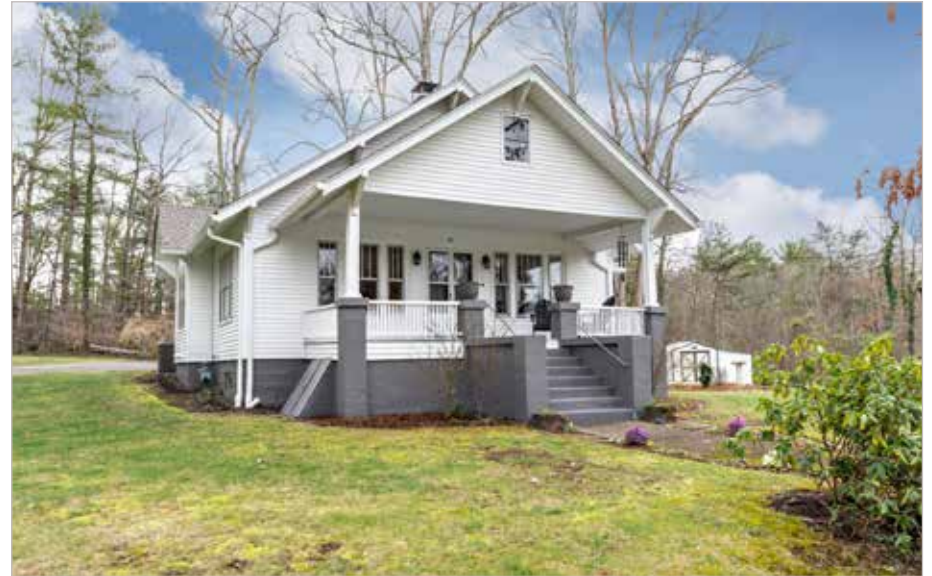
Low-Maintenance Exterior (Original Wood Siding Underneath Vinyl)
