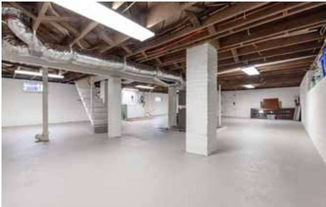
Dry Basement with Space for Storage or Workshop
