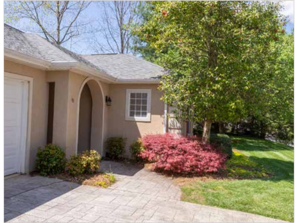
2020 Architectural Shingle Roof
