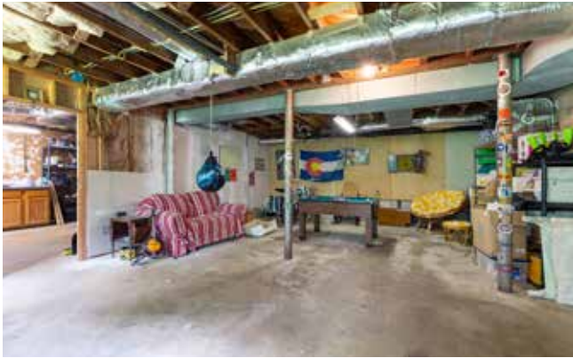
Bonus Space in Basement
