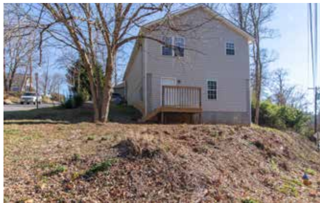
Walk-Out Basement is Ready to Finish
