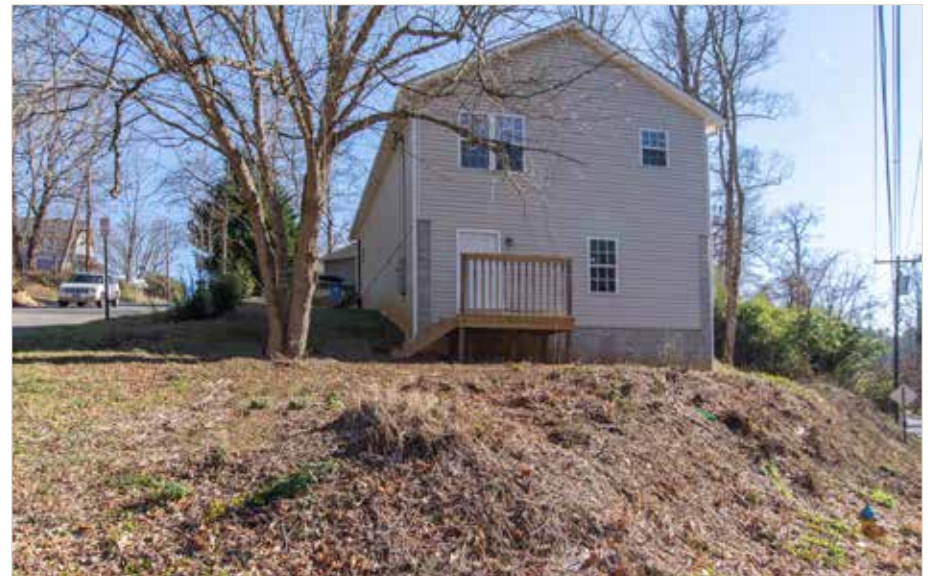
Entrance to Walk-Out Basement
