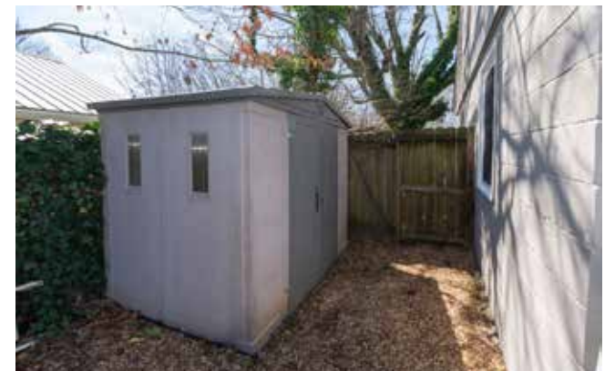
Convenient Storage Building for Lawn Equipment
