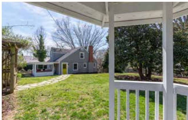
Side Entrance to Kitchen
