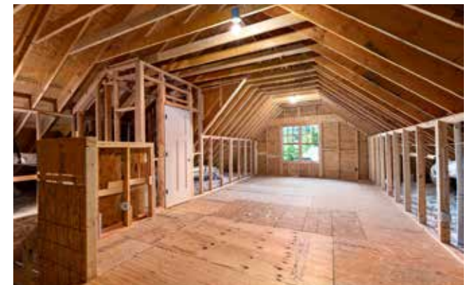
Framed-in, Wired Attic, Ideal for Future Bonus Room
