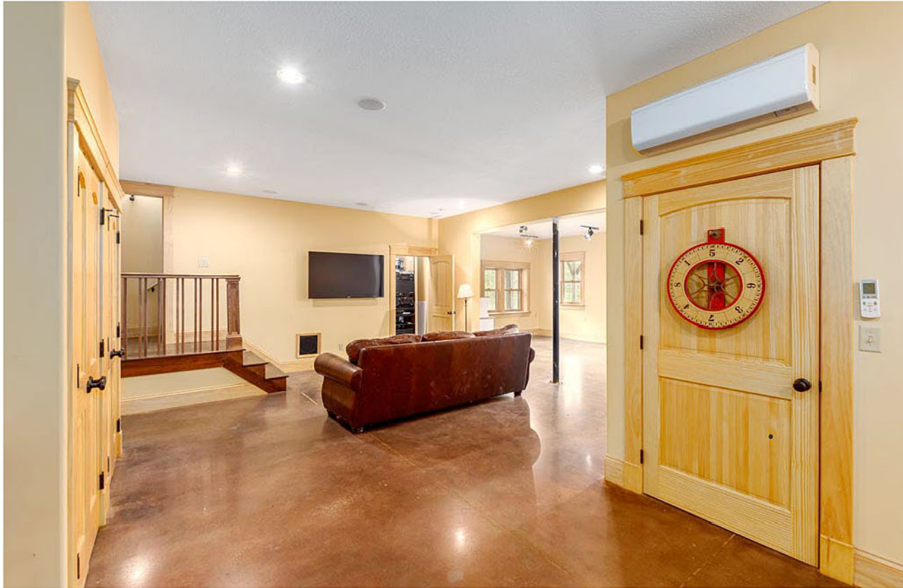
Lower Level - Radiant Concrete Floors
