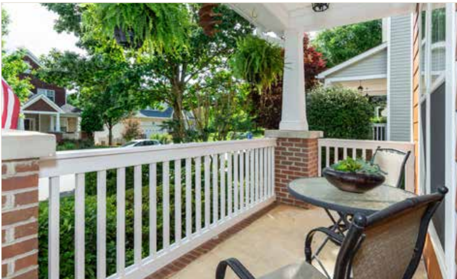
Covered Front Porch
