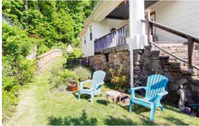
Stone Foundation Wraps the Home
