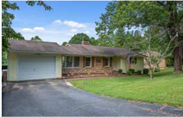
Upper Level Garage
