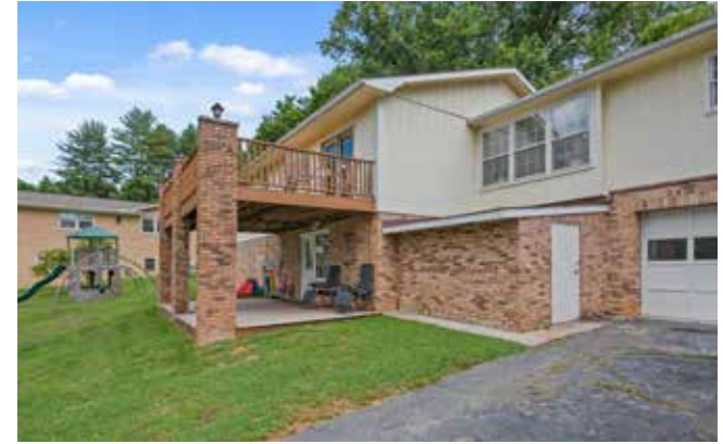
Lower Level Garage
