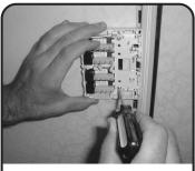
A surface mount box can be mounted with the two 6-32 x 1/4 inch screws provided.
