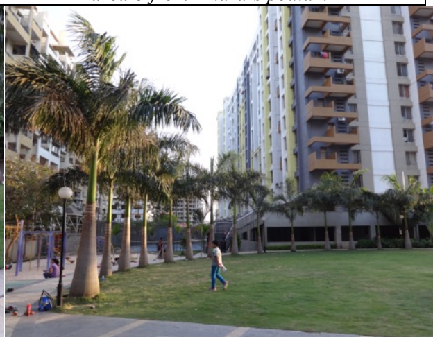
Figure 6.6.k. View of Central lawn-4 looking towards Phase-2 residential buildings at Dhara
