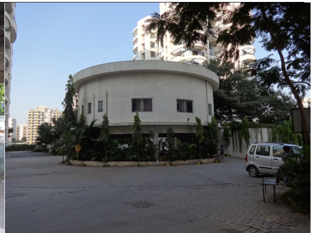
Figure 6.3.n. Outside view of Semi-open space below society office-5 at Keerna
