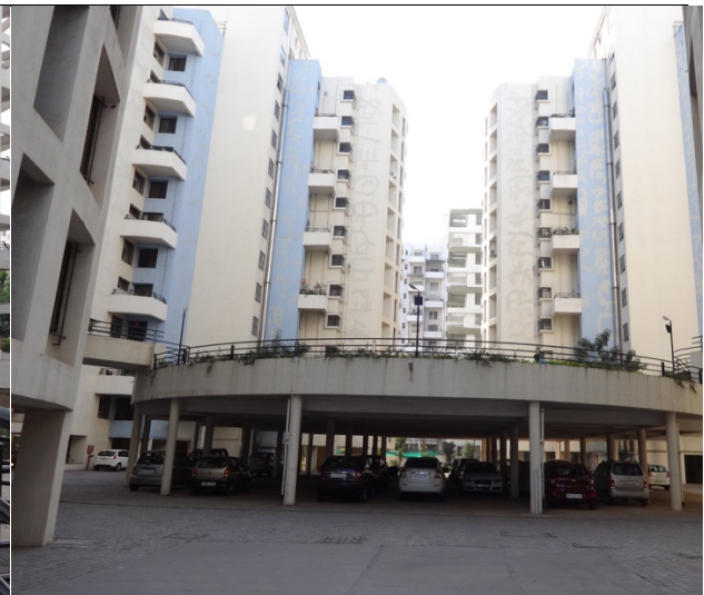
Figure 6.3.h. View of Older children's play area-2 from ground level at Keerna
