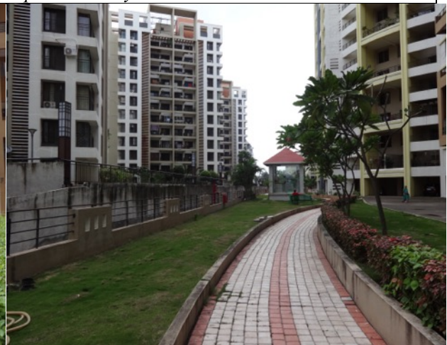
Figure 6.6.n. Walkway adjoining Green pocket space-6 on Dhara's podium
