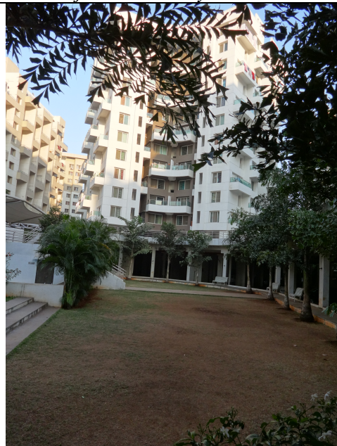
Figure 6.2.h. View of Central lawn with clubhouse and amphitheater-2 at Ambar
