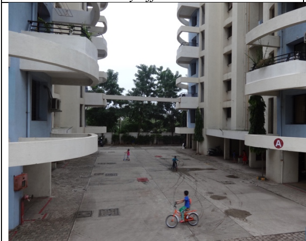
Figure 6.3.o. Parking area-6 and driveway at ground level between A and D buildings at Keerna
