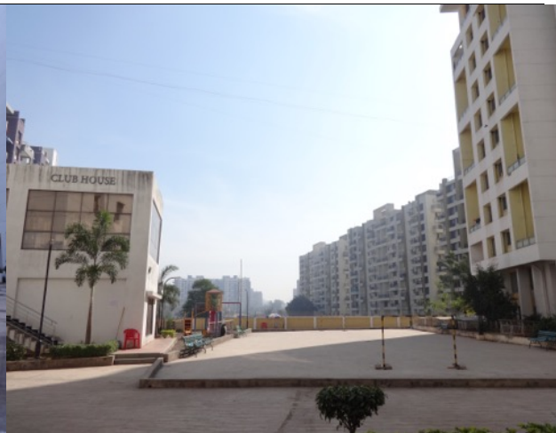
Figure 6.5.l. View of Concrete playing field-5 and clubhouse at Shakti
