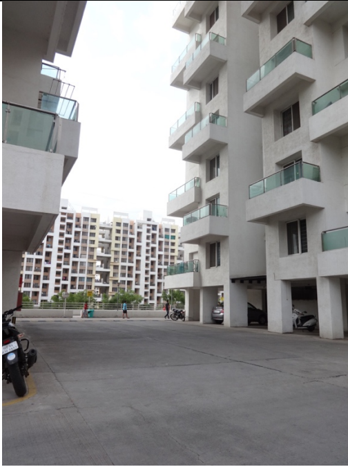
Figure 6.2.k. Driveway between buildings-4 on podium at Ambar
