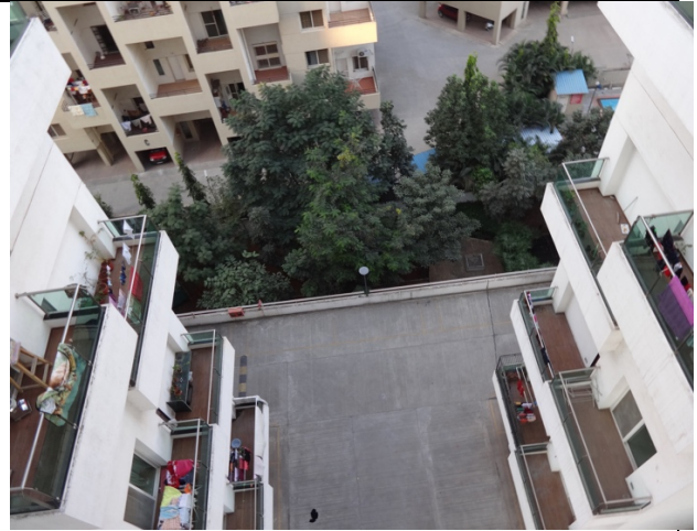
Figure 6.2.l. Top View of Driveway between buildings-4 at Ambar
