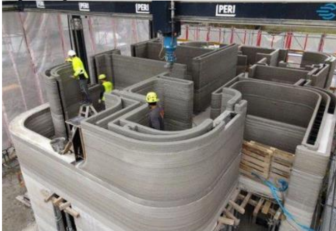
Fig 8. A 3D machine printing a house
