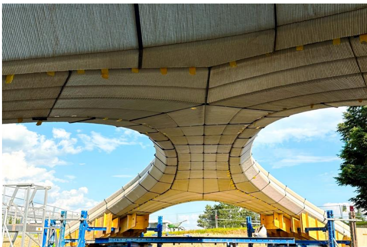
Fig 7. The future of 3d printed bridges (New Civil Engineer)
