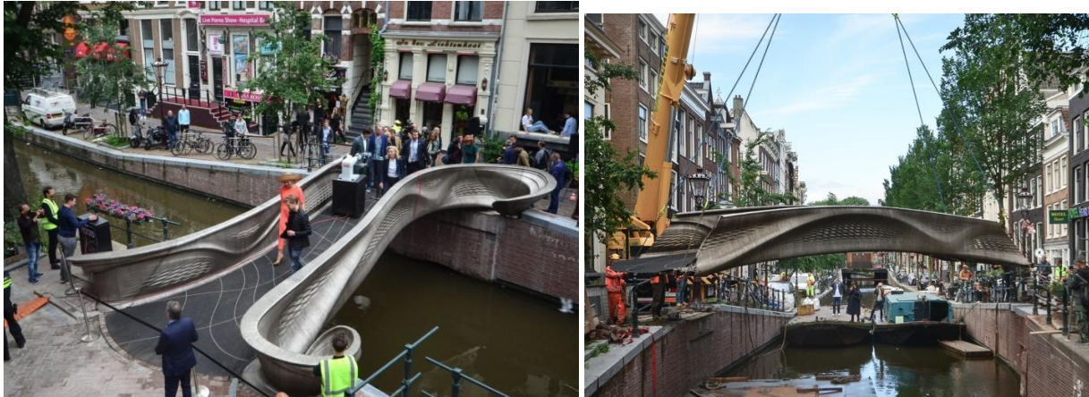
Fig 8. Pictures showing the first 3d built bridge
