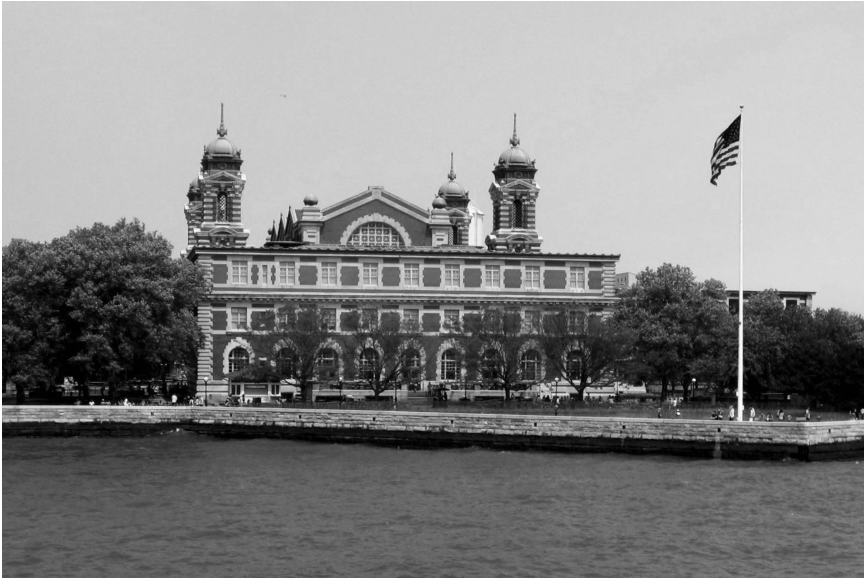
Figure 17.3 A triage centre for immigrants, Ellis Island was also meant to impress newcomers with its grand architecture.
