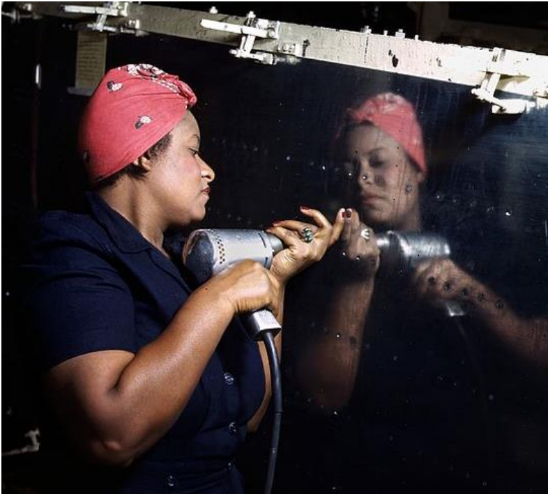
A real-life "Rosie the Riveter" operating a hand drill at Vultee-Nashville, Tennessee, working on an A-31 Vengeance dive bomber, by Palmer (1943)
