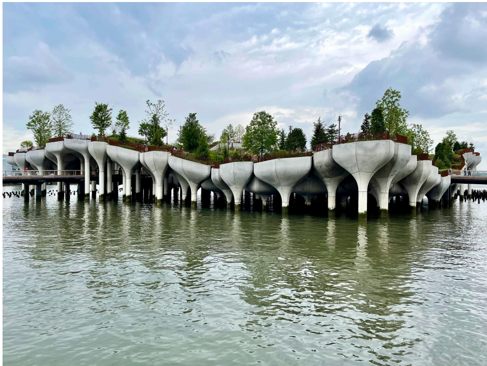
Figure A4 Little Island . Artificial island park supported by distinctive tulip-shaped concrete columns above the Hudson River.
