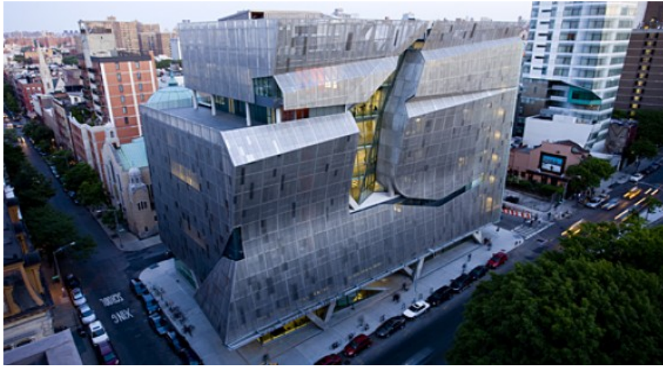
Figure A3 Cooper Union New Academic Building . Known for its perforated stainless-steel façade and central atrium designed to promote airflow and natural light.
