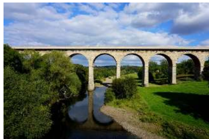
Figure 2.11.1 "bridge" barnyz is licensed under CC BY-NC-ND 2.0
