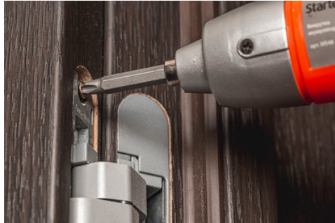
Figure 2.7.1: "Close-up, electric screwdriver secures the door hinge" by Marco Verch is licensed under CC BY 2.0.
