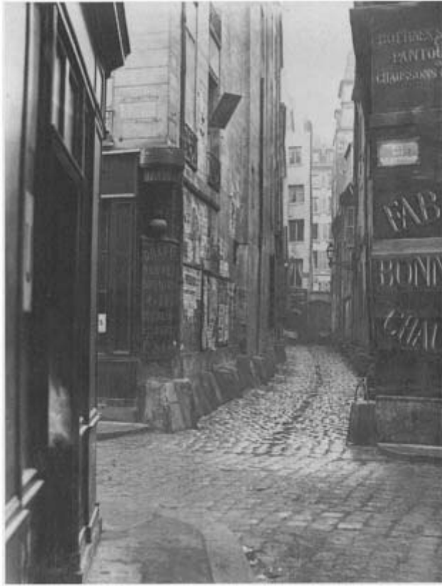
FIGURE 88 Most of Marville's photos of old Paris seem to have been taken shortly after a rain shower, for there are invariably runnels of liquid in the street. But these runnels are, for the most part, indicators of raw sewage. Much work was needed to remedy this unhealthy situation.
