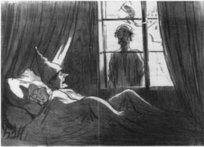
FIGURE 47 The demolitions affected everyone. In this Daumier rendition (1852), a workman is telling a bourgeois couple to hurry and get up, because they are next in line for the pickax.
