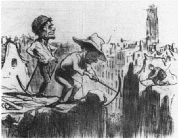
FIGURE 51 Construction workers were everywhere after the demolitions truly got going. Here Daumier has two workers speculate that the reason the Tour St. Jacques (to this day an isolated landmark in the city) is being left standing is because it would require an ascent by balloon to demolish it.
