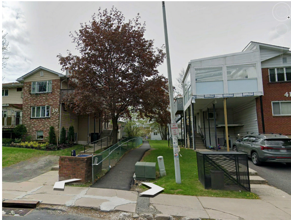
Constructed pedestrian sidewalks in the village. Source: Google Earth Pro.
