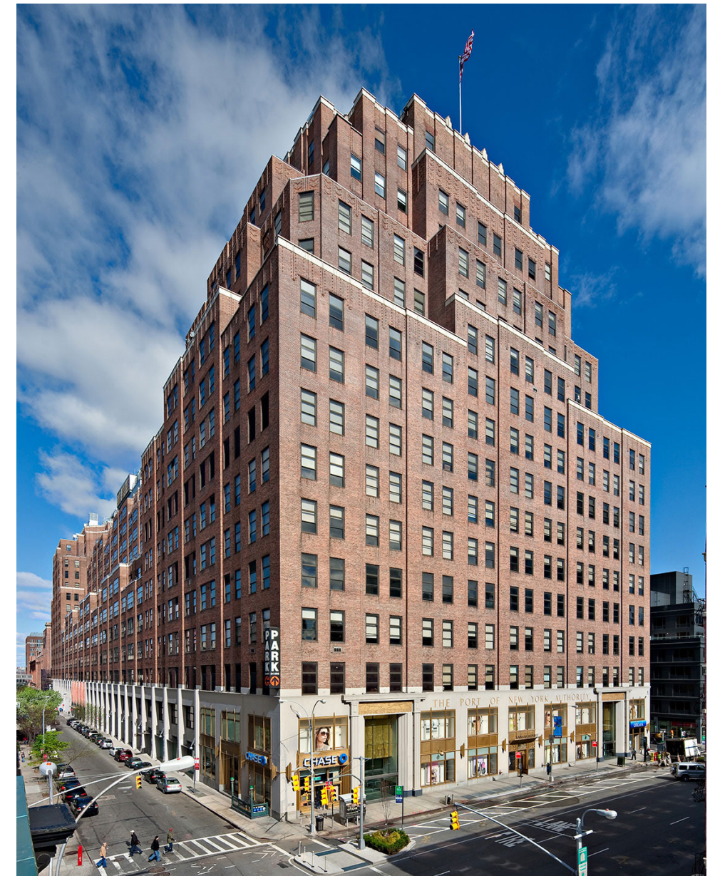
Equinix NY9 Data Center at 111 8th Ave New York, NY 10011.
