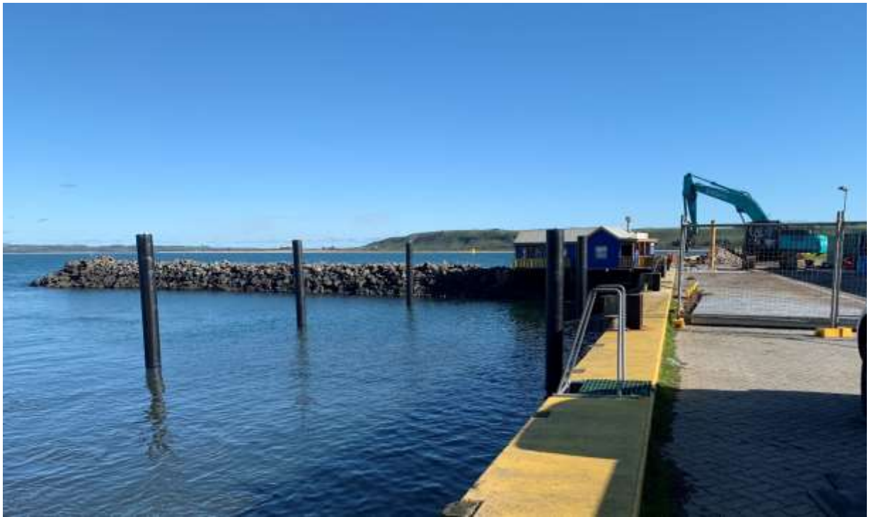
Above: Pylons are being driven in readiness for a floating pontoon that should be finished by the end of the year. Work is being undertaken by TasPorts.
