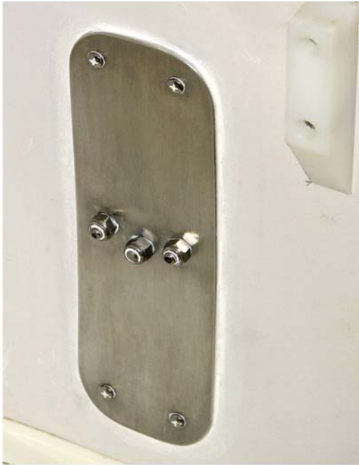
Load-transferring/Backing Plate in Bathroom/Shower Area
