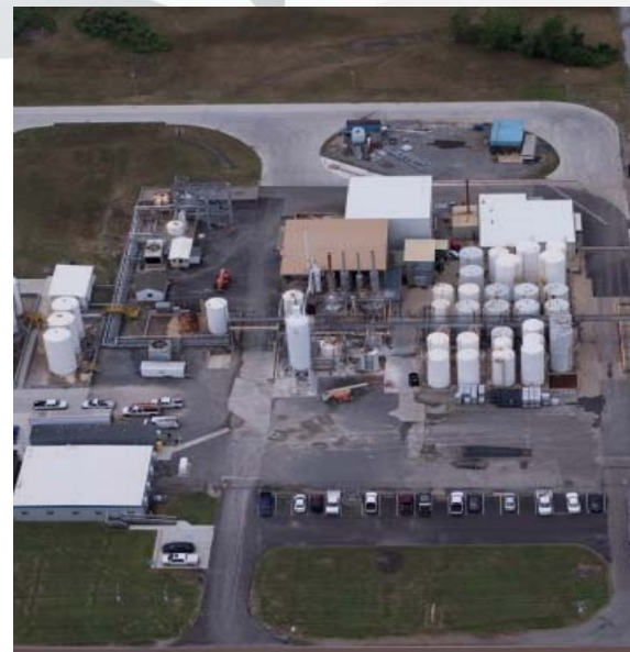
West Memphis Brominated Clear Brine Fluids Manufacturing Plant
