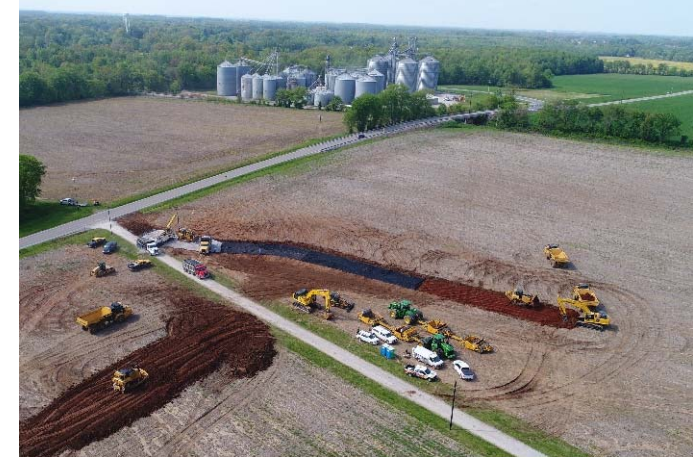
Beginning to break ground in Guthrie, Kentucky
