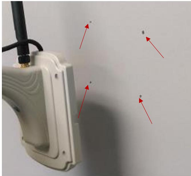
*Figure 1: Make four markings for the screws.*
