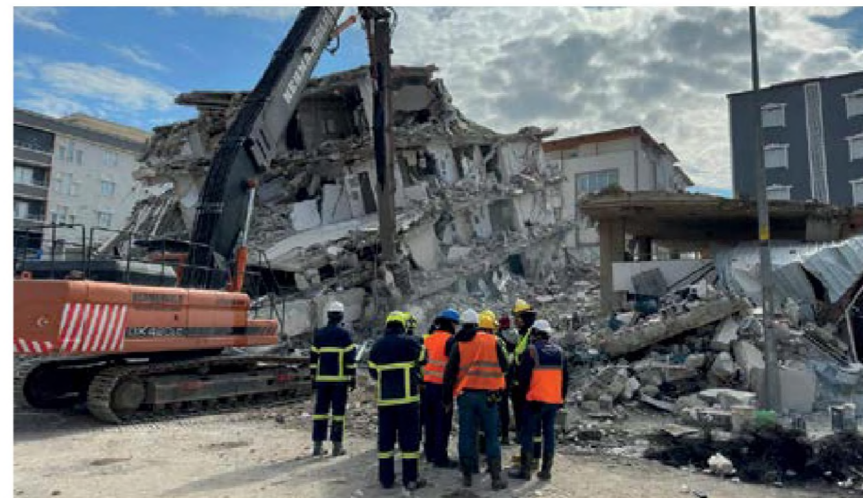
Kurdistan Region crew removing building rubbles in the aftermath of earthquakes in Turkey.
