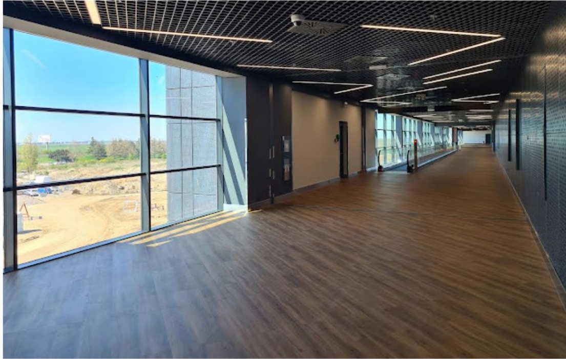
New floor (arrivals corridor)
