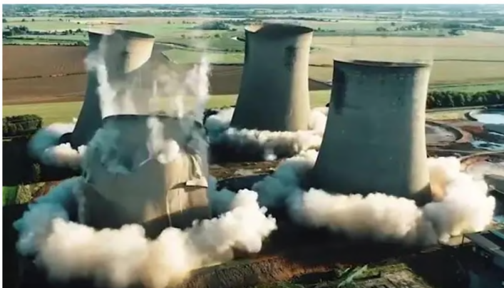
Watch moment 4 power station towers are demolished in huge explosion
