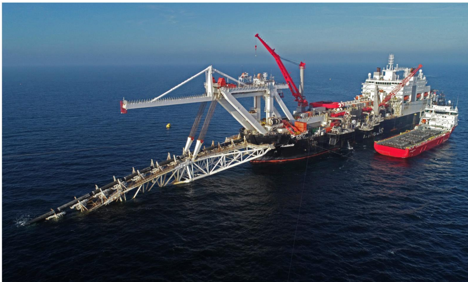
Laying of Nord Stream Two pipeline (Source: AFP)
